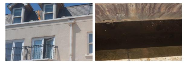
We are aware of previous leaks occurring in similar locations on this property, and water ingress could be entering either from a failed EPDM membrane lining the box gutter, or down from the slated roof mansard, weeping in behind the EPDM membrane as it laps up the roof slope.
