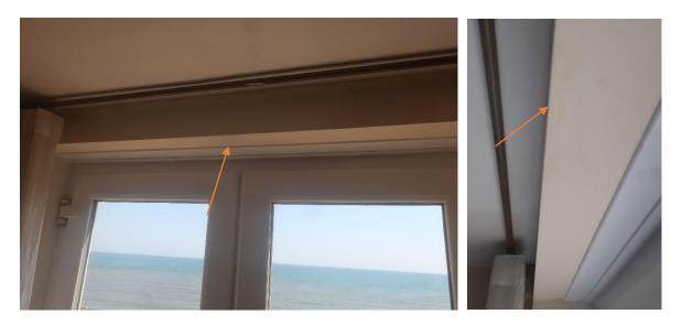
On inspection, there is a small area of paint that has peeled and I was shown copies of photos indicating damp staining.
