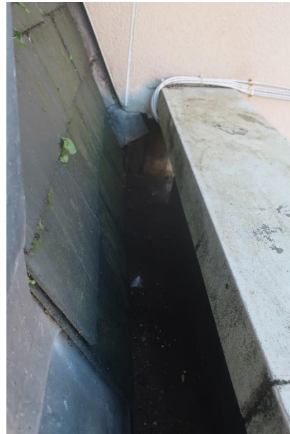
Box gutter adjacent flank wall
