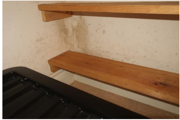
Rear wall of fitted wardrobe
