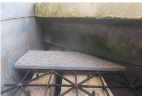
Whilst we could not lift all the decking to fully inspect the lead sheet roof, in the areas exposed it was not defective, plus the dampness noted in the ceiling of the wall below is positioned further out within the thickness of the wall itself, as opposed to directly beneath this bay roof.
