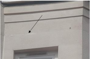
With most weep holes now no longer being present, there is a possibility that the cavity trays are filling up and overflowing, especially if they are not proprietary trays with corner upstands, as buildings of this age typically had sheets of polymer DPC used to act as the tray.
