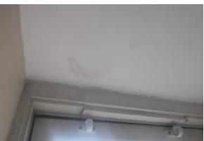
To the left-hand splayed reveal when looking out, paint blistering also extends down the left-hand reveal of the window which, again, is lined in plasterboard.
