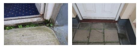
The frame to the entrance door is rotting and water could obviously penetrate through where the asphalt stops underneath the door threshold.
