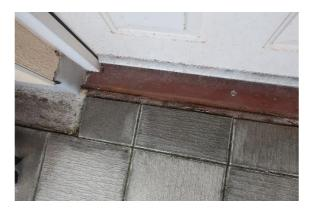
In addition, the wall area adjacent the stairway door, the asphalt is starting to pull away and is split in the corner where the stairwell meets the wall of Flat 21, and all these areas require re-sealing, ideally having a lead flashing over.
