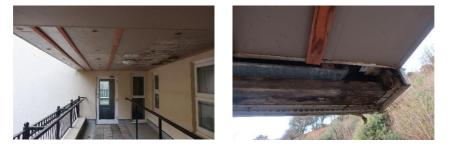
This ceiling soffit forms the underside of the balcony slab which accesses Flats 20 and 21 and we understand from speaking with the Lessee in one of the Flats, that previous works have been undertaken to this balcony, with a rainwater gulley being installed at a later date, as the balcony was ponding heavily due to it not being laid to adequate gradients initially.
