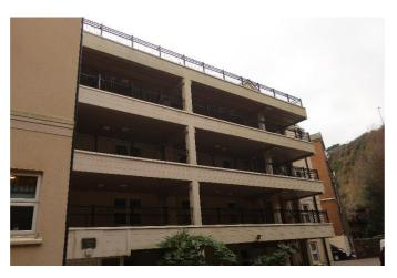
The problem in relation to the balconies is apparent on the rear elevation only as the rear elevation is provided with a central stairwell and open balconies and entrance landings being provided to give access at each floor level.
