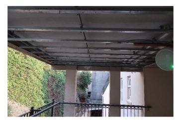
It does therefore appear that water has been penetrating down through the perimeter walls, but moisture is also travelling across in various areas of the balcony, affecting the ceiling support grid.
