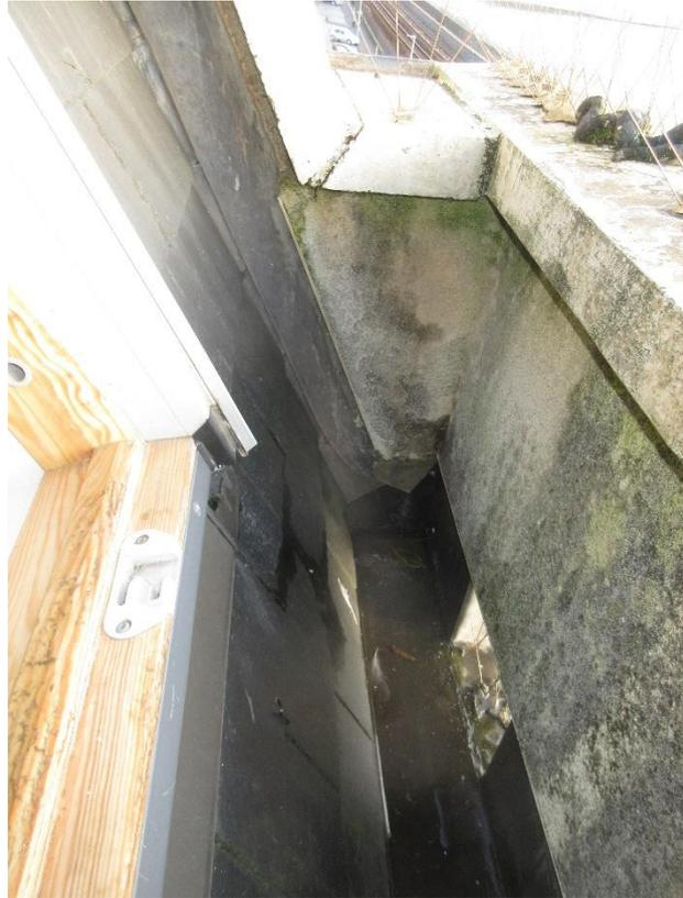
Fig.3 Parapet box-gutter lining appears to be partially collapsed and leaking, saturating the concrete floor of the flat.
